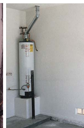
Garage installation of water heater
