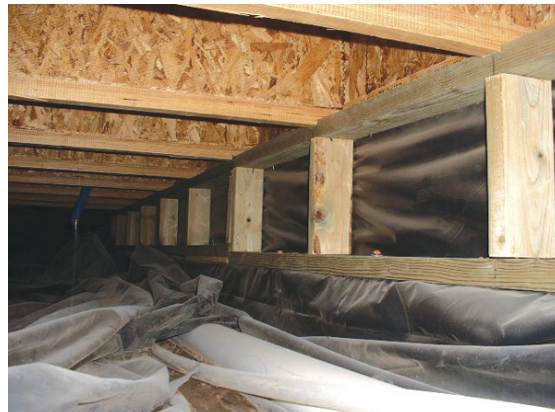
Figure SC-7: Conditioned crawlspace
