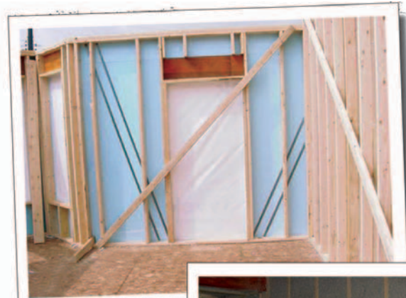
Continuous rigid insulation for thermal break
