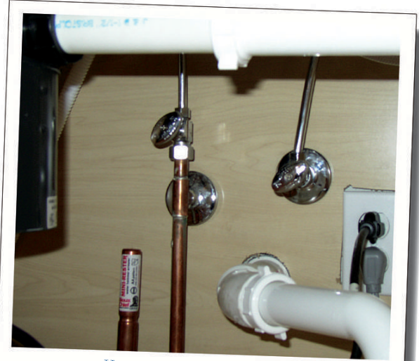
Hot and cold water shut-offs under the kitchen sink
