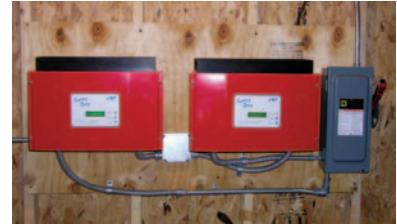
The inverters are located in the garage
