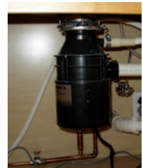
Garbage disposal located under kitchen sink
