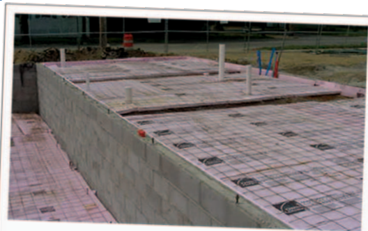
Slab-on-grade insulation
