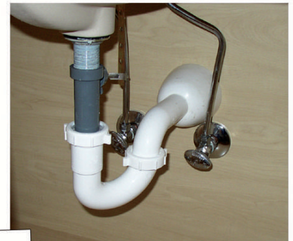
Hot and cold water shut-offs under the bathroom sink
