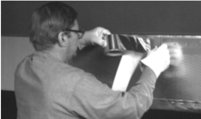
Fig. 25. Seams and joints of faced boards are sealed with glass fabric and mastic or with pressure sensitive tape.
