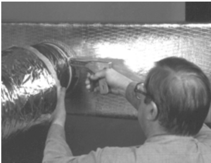
Fig. 31. Applying plastic closure strap to flexible duct
