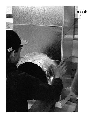
Applying fabric mesh before spreading mastic provides this large joint with a strong and airtight seal. Airtight ducts are one of the key ingredients to a comfortable and energy-efficient home.
