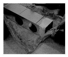
Duct trunks are easier to insulate before they're installed. After ducts are installed, hangers and other obstacles can make installing insulation difficult.
