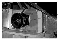
Return plenum temporarily disconnected and opening to air handler blocked here.
