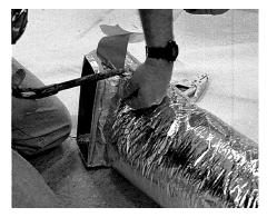
Making a tight seal between the flex-duct's insulation and the boot's insulation is important for preventing condensation from damaging the insulation during the cooling season.
