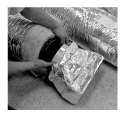
Insulating boots and fastening them to flex-duct is another effective prefabrication that is easier to perform outside an attic or crawl space.
