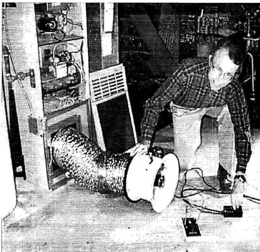
Figure 2 Duct Blower at fan access opening with use of cardboard "custom-cut" mounting.
