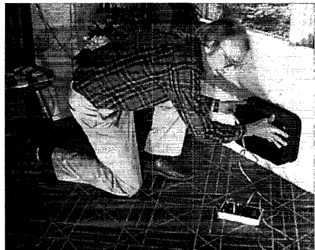
Figure 5 Pressure pan used to determine duct leakage in individual duct branches
