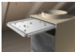
1. The polyester filter removes larger dust particles
